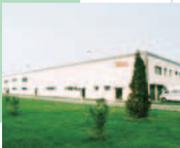
Tianjin Stanley Electric Co., Ltd.
